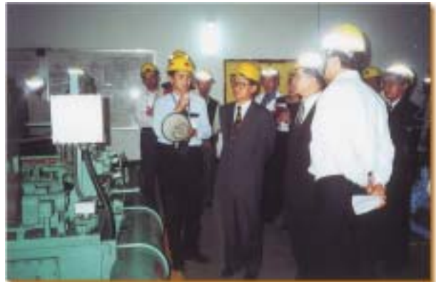
Members of the Control Yuan make a circuit supervision and inspection of the Yu Cheng Pumping Station of Taipei City Government.
